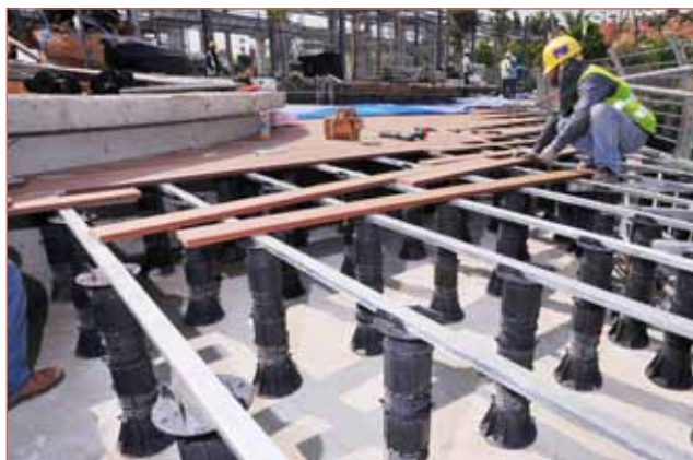
VersiJack® provides stable support for installation of decking
